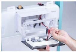
Route the red 12V cable to the cistern via a conduit or sleeve.
