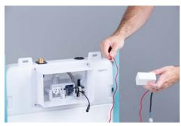
o ------ Install the supplied transformer in a suitable and accesible location in accordance with the local electrical bylaws.
